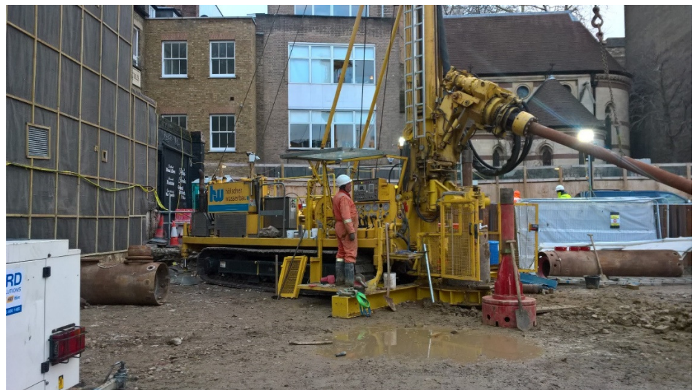
Drilling operations over the 1 st Borehole.
